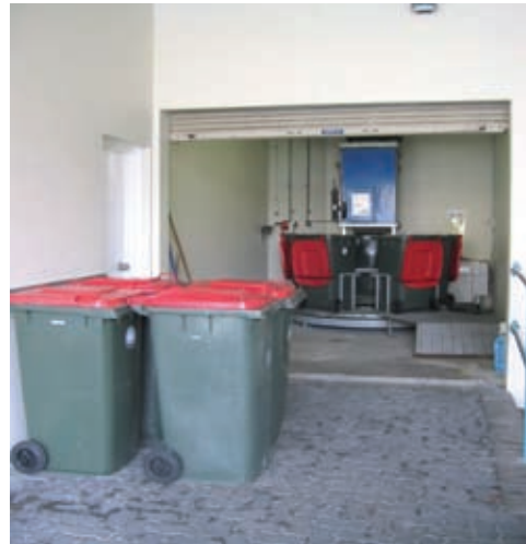
Rear loading dock and waste compactor
