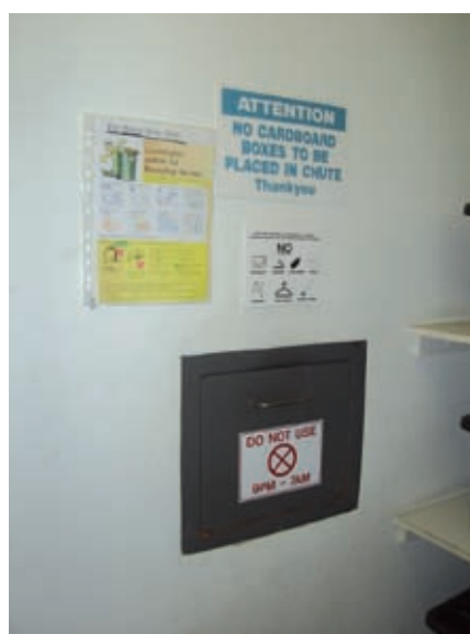
Signage in service compartments of the tower
